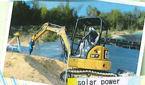
solar power installation work
